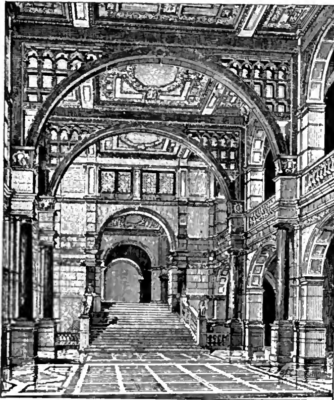
FIG. 96.—Staircase, Imperial Institute. (Collcutt.)
